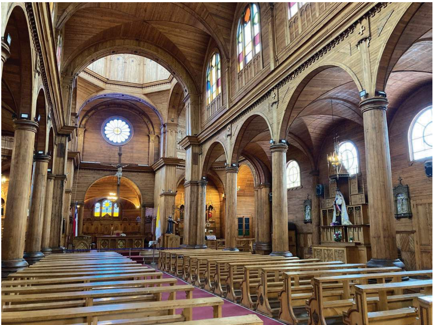
Fig. 8. San Francisco church, on the Plaza de Armas in Castro, the main Catholic temple in the capital of the Province of Chiloé. In the structures, wood from the area was used, such as Alerce, Coigüe, and Guaitecas Cyress. The interiors are made of Rauli (imported from the mainland) and Olivillo. The roof, front, and external linings are made of galvanized iron sheets.
