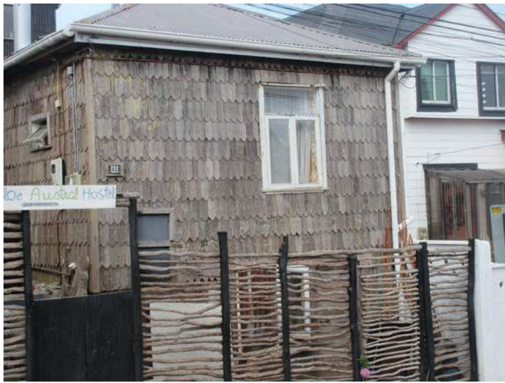
Fig. 7. Example of wooden shingles on a house in Castro lakes or lagoons (Fig. 12). The construction of these overwater bungalows and structures in Chiloé originated during the 19th century when the whole area underwent a great commercial expansion, especially in the fishing industry, which allowed fishermen to live by the water and moor their boats next to their homes. In addition, since it was public land, the fishermen could
